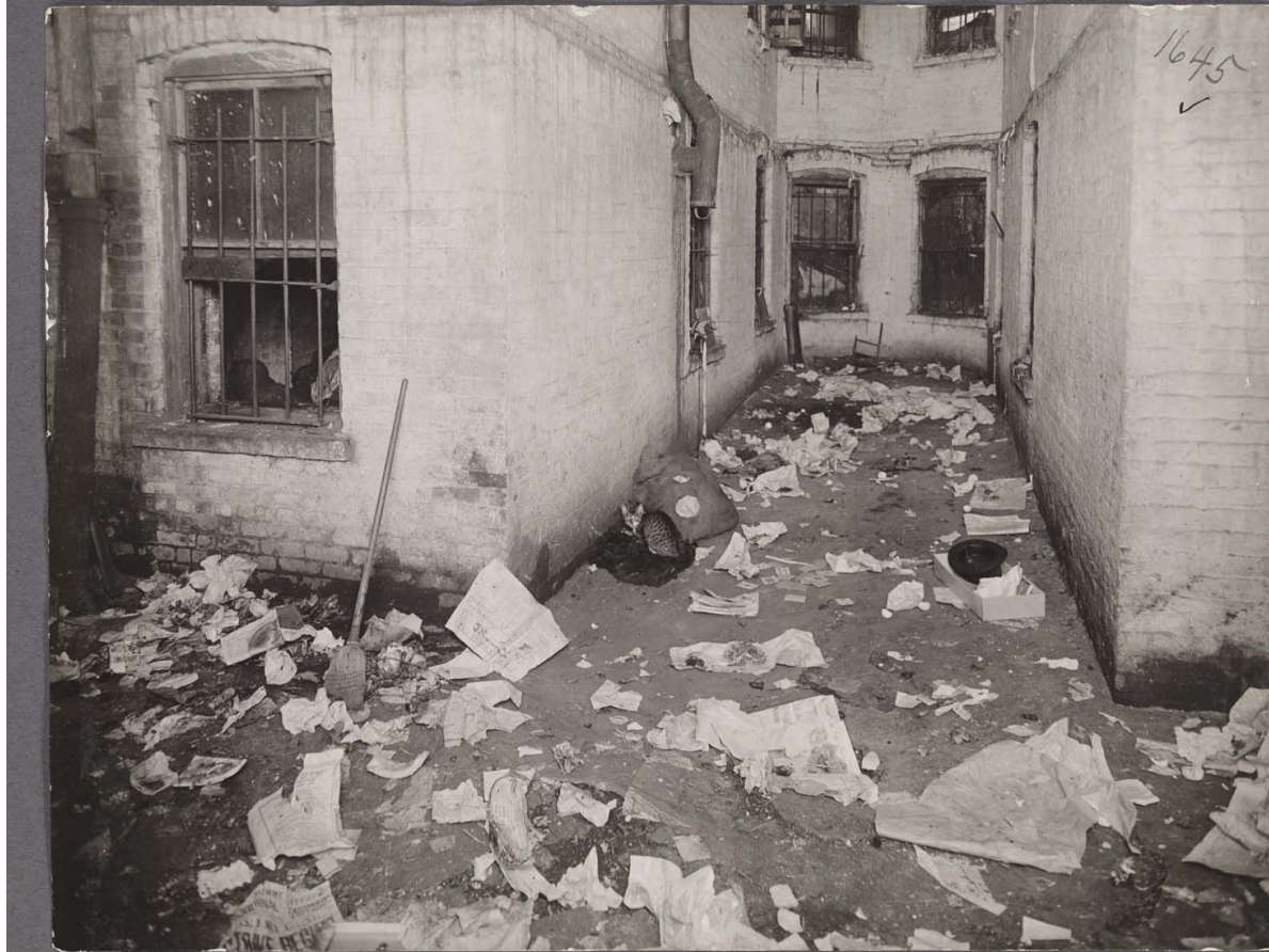
Garbage in an air shaft
